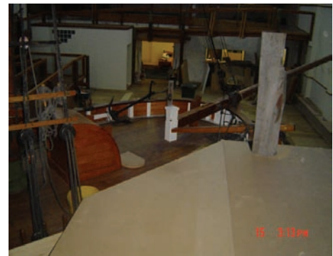
View from the wharf after one days construction-top job-Project Hahn.
